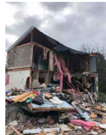
The Kline's home after the fire
